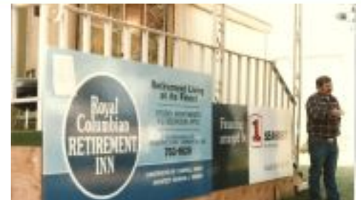
The temporary marketing building while under construction.
